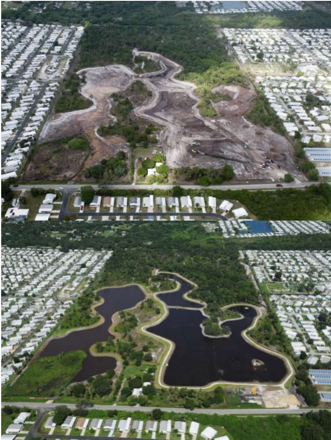
Figure 80: Powell Creek Filter Marsh during construction and before planting
