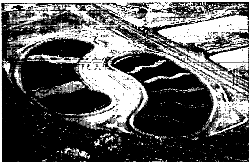
The Hayfield Site demonstration wetland at Tres Rios west of Phoenix, Arizona, includes two cells with variable numbers of deep water zones to test their effect on hydraulic efficiency and wildlife habitat.
