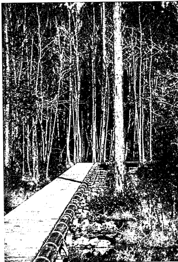
Gated pipes on raised boardwalks allow access to more than 600 acres of treatment area in the Vereen Natural Treatment Wetland in South Carolina.
