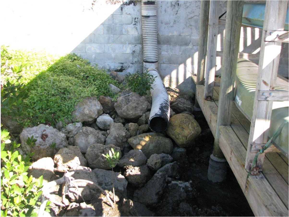
Figure 62: Outfall pipe into the Harbor Marina. This is an area of sediment deposition within the basin.
