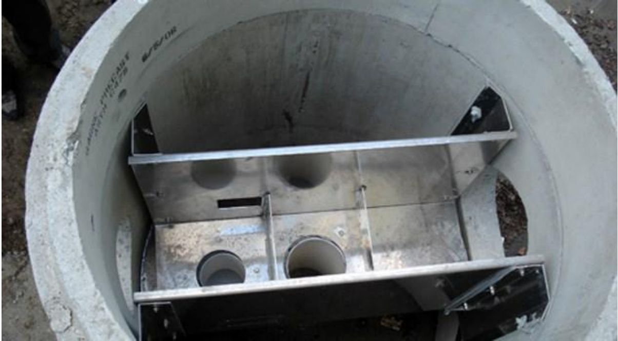
Figure 52: Installed Vortsentry HS unit
