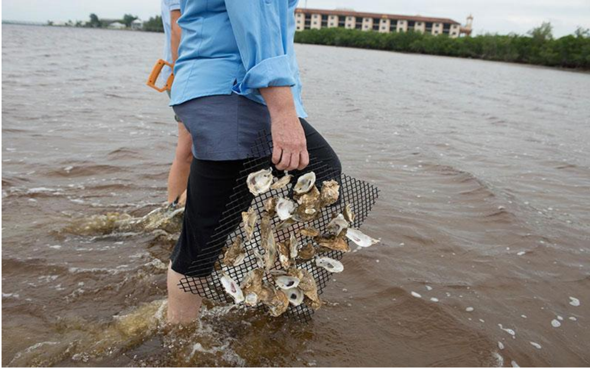
Figure 10: Citizen Volunteer deploying an oyster screen into shallow waters of the Peace River for a living shoreline project, City of Punta Gorda.
