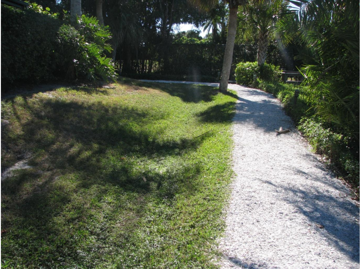
Figure 55: Existing swale at south end of South Cove Harbor. This is recommended to be replicated parallel to Little Sarasota Bay along all of South Cove and Far Harbor behind the mangroves and marsh living shoreline. Drainage from land surfaces would be directed in other swales into this coastal swale system.
