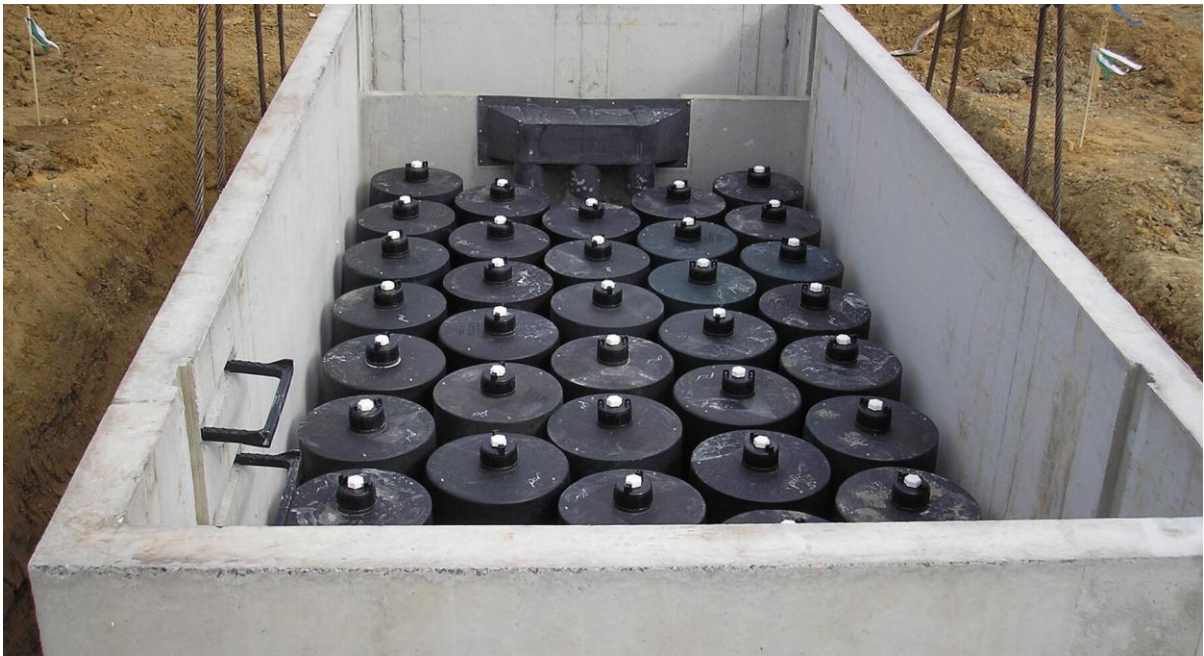
Figure 45: StormFilter System installed in a vault.
