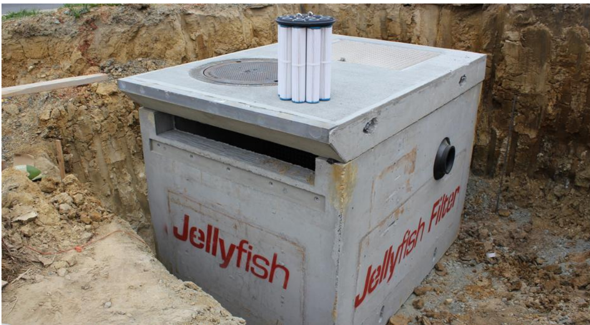
Figure 49: Jellyfish Filter Vault Installation
