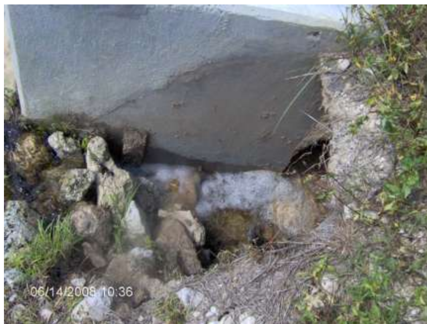
Figure 26: Erosion around the southernmost weir at San Carlos Estates. Source 2008: Exceptional Engineering, Inc
