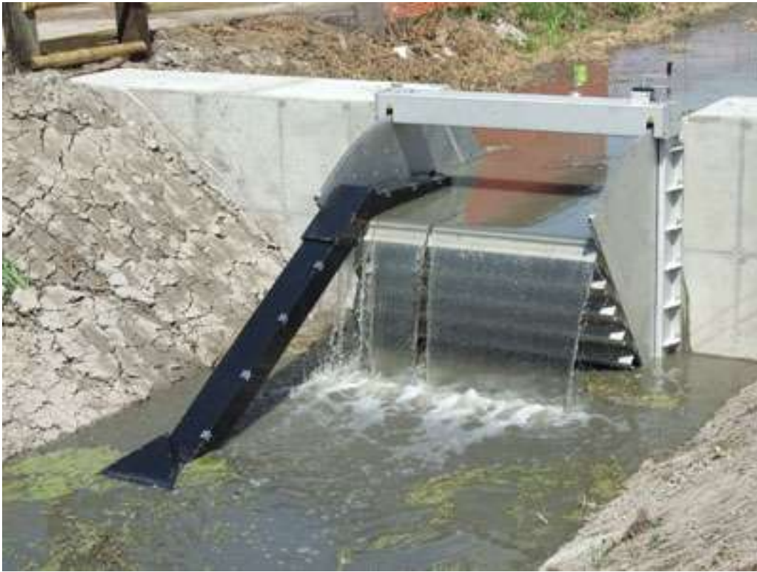
Figure 28a; Other adjustable weir designs with a fish chute.
