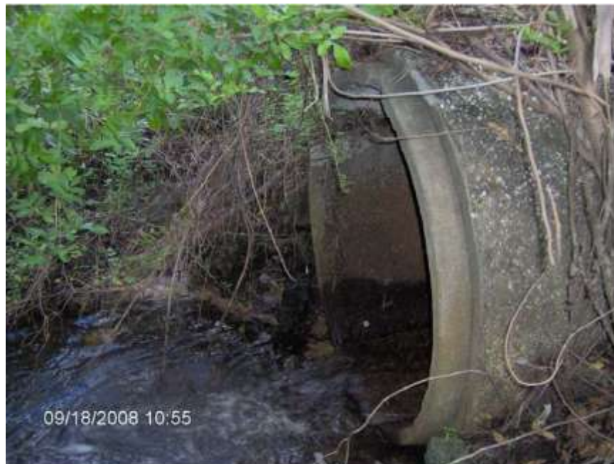
Pic 23. 48" RCP at FPL easement
