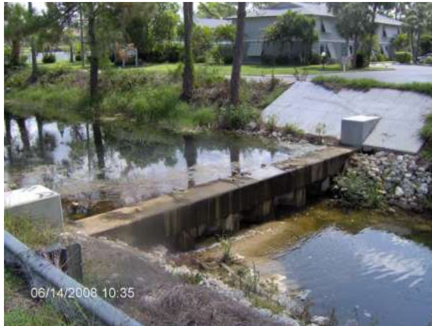
Figure 25. San Carlos Estates southernmost weir. Note: flow from erosion. Source: 2008, Exceptional Engineering, Inc
