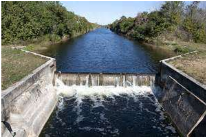
Figure 28a; Other adjustable weir designs with a fish chute.
