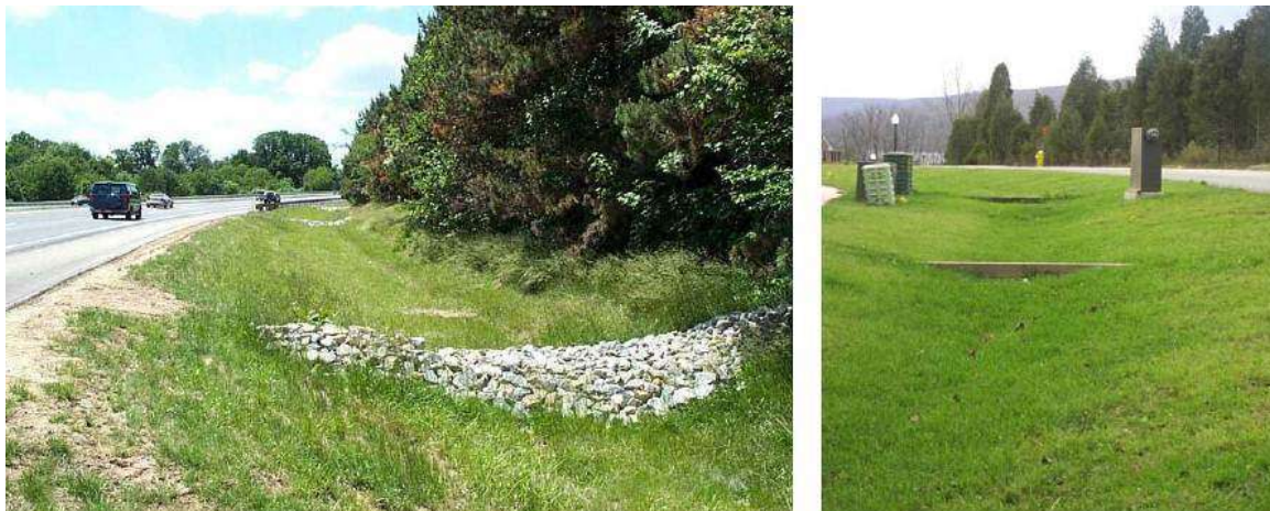
Figure 31: Example design of a grassed swale for roads leading to Strike Lane.
