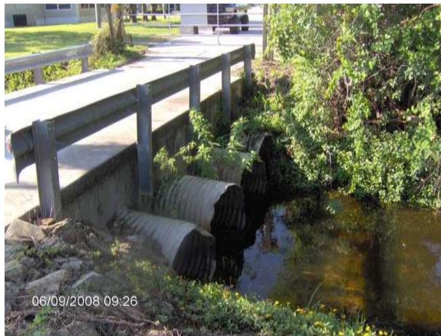
Pic 14. Imperial Harbor CMP pipe crossing. Figure 25: Pic 14. Imperial Harbor CMP pipe crossing. Source 2008, Exceptional Engineering, Inc
