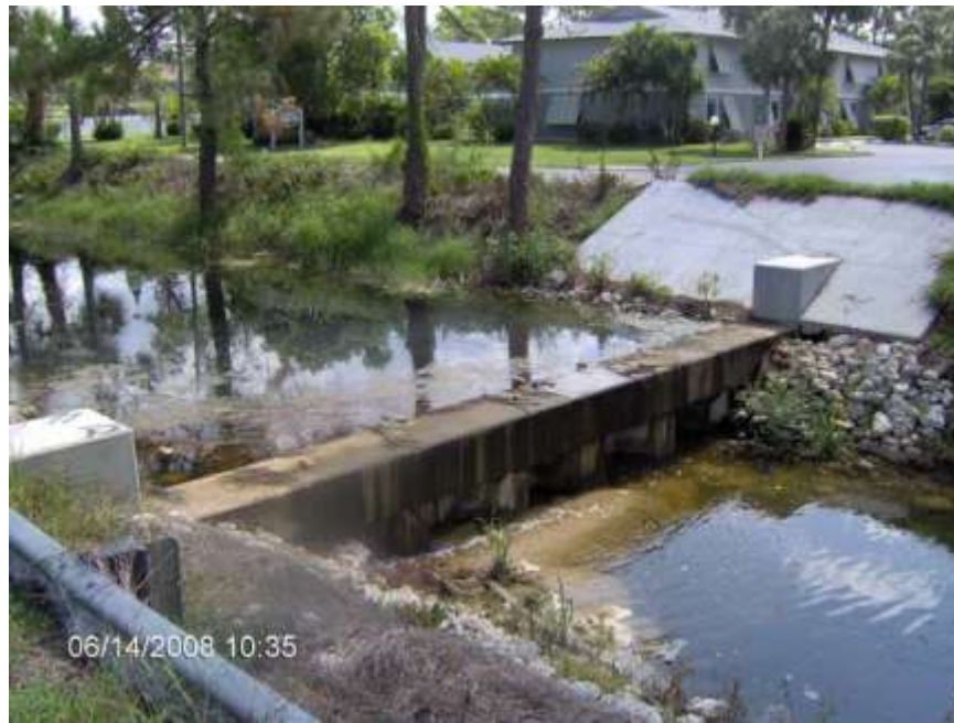
Figure 10: San Carlos Estates southern most weir. Note: flow from erosion. Source: 2008, Exceptional Engineering, Inc
