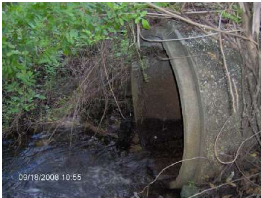
Pic 23. 48" RCP at FPL easement
