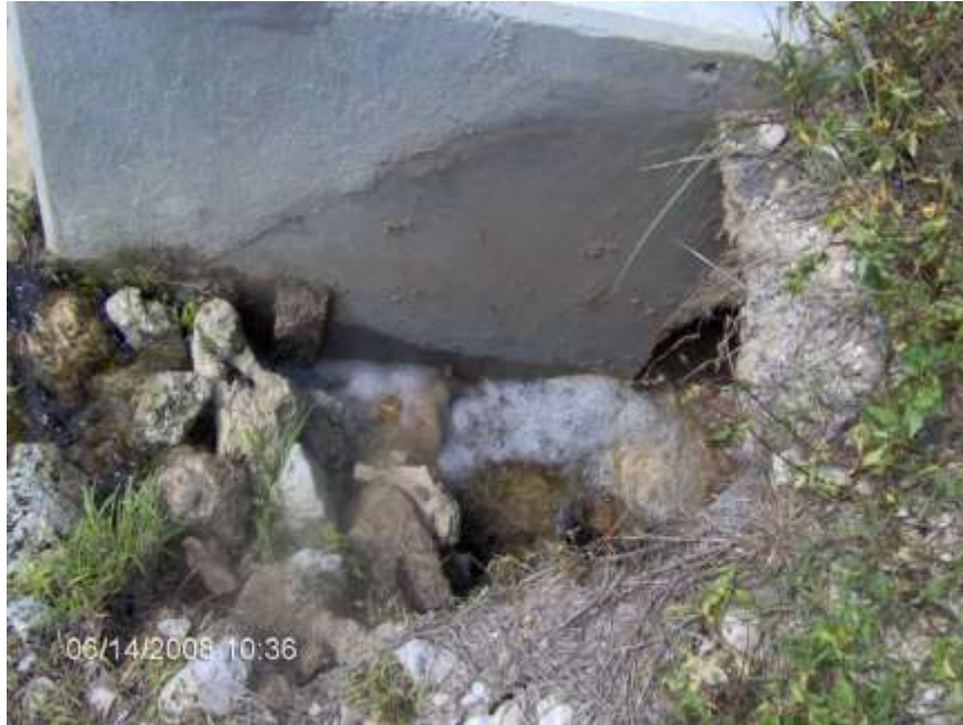
Figure 11: Erosion around the southernmost weir at San Carlos Estates. Source 2008: Exceptional Engineering, Inc
