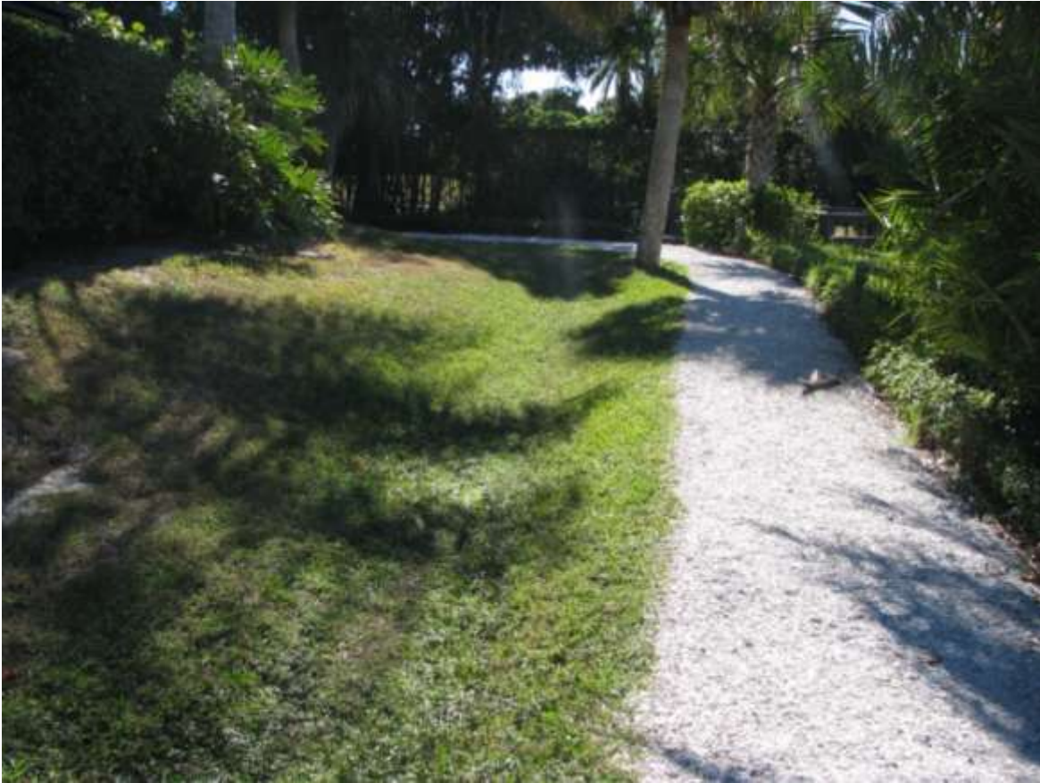
Photograph 2: Grassy swale system typical of stormwater conveyance in Bayhouse Area, Building #1.
