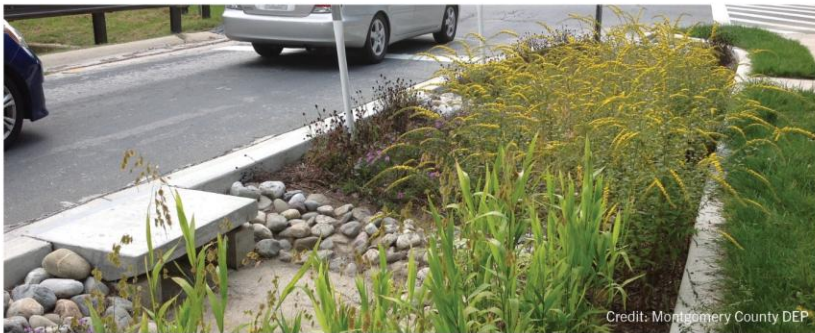
Credit: Montgomery County DEP
