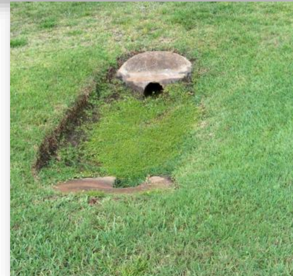
Examples of private stormwater systems (Top: wet detention system; Bottom: swale)
