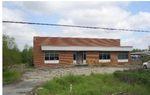
Deteriorating residential and commercial areas
