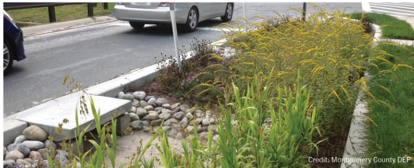
Credit: Montgomery County DEP
